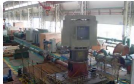
PN.8 Circulation Water Pump Testing
