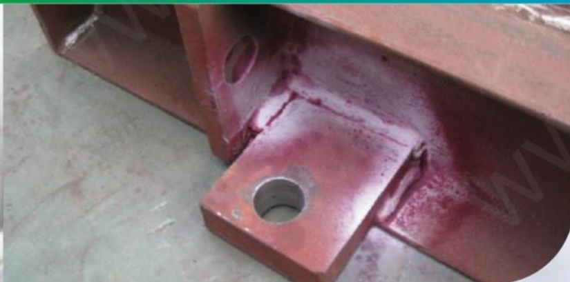
PT: Liquid Penetrant Inspection / Welded Baseplate
