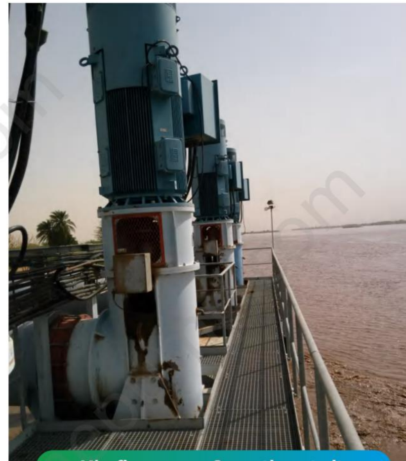
Mix-flow pump Operation at site
